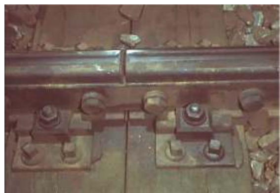
On-board visual inspection system stores images of tracks and turnouts
