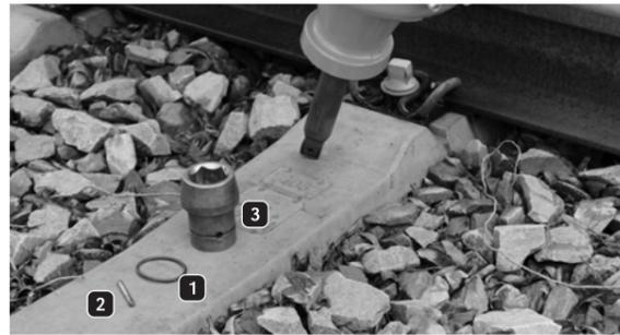
Figure 30: Replacing the socket wrench insert
